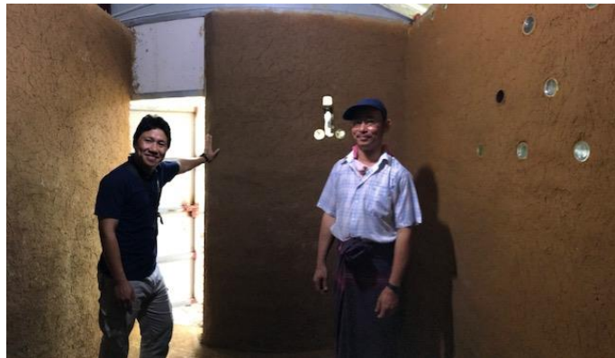
Figure 8. Boonsong (ECHO Asia staff member) inspects the new earth block seed storage room at the Sustainable Agriculture Training Center.
